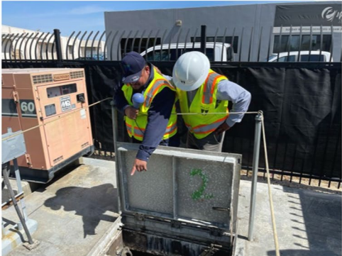
Photo 10: District staff inspecting wet well at station.
